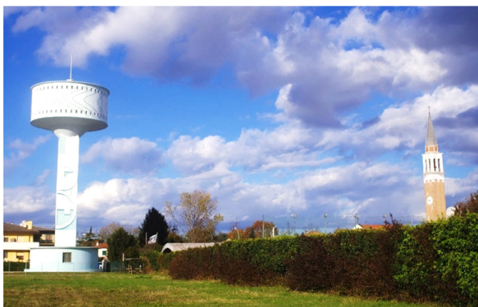
Fig. 17. The water tower seen from the south with the bell tower of the Borbiago church.
