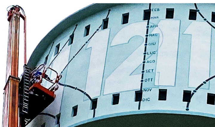
Fig. 10. Crane-mounted 'cherry-picker' work platform.
